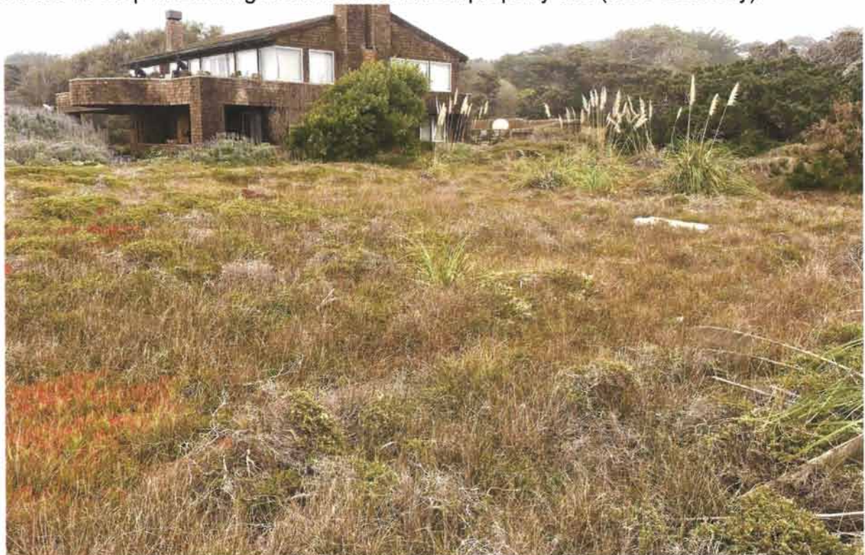
Photo 2. Step 2. Looking north from southern property line (near driveway).
