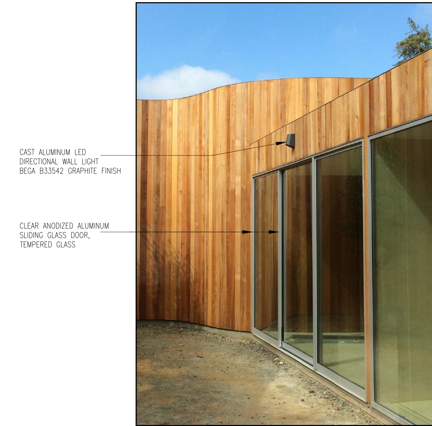
TYPICAL EXTERIOR SLIDING GLASS DOOR
